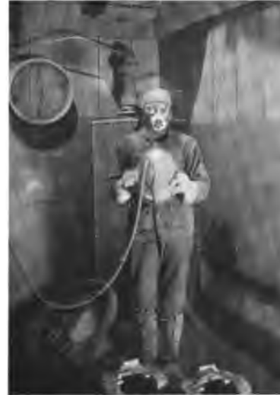
Fig. 2. Sand-Blast Operator. (American Steel Foundries Company.)
